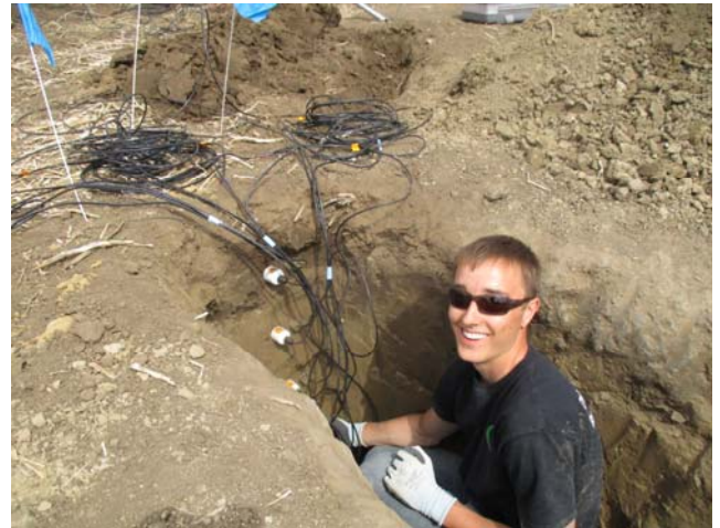
University of Calgary student installing soil moisture sensors at the GRIP site near Lethbridge.
